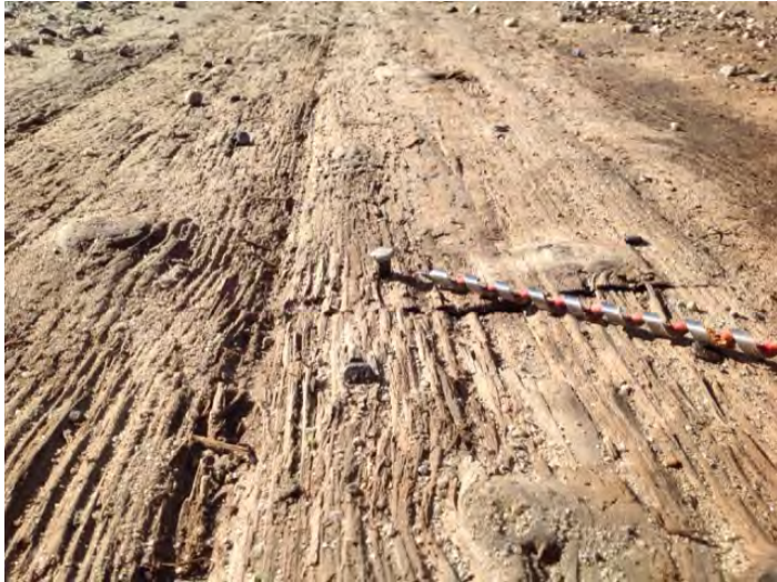
nails starting to protrude
