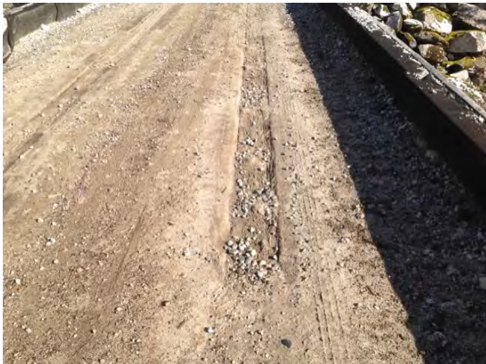
wheel path decking wearing
