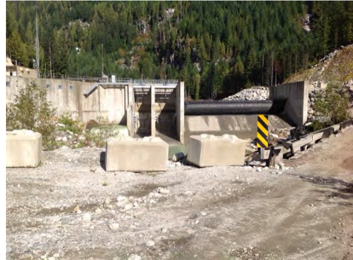
dam immediately upstream from crossing
