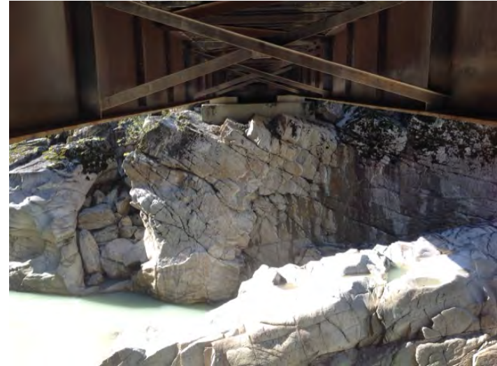
Right Bank Abutment when facing downstream
