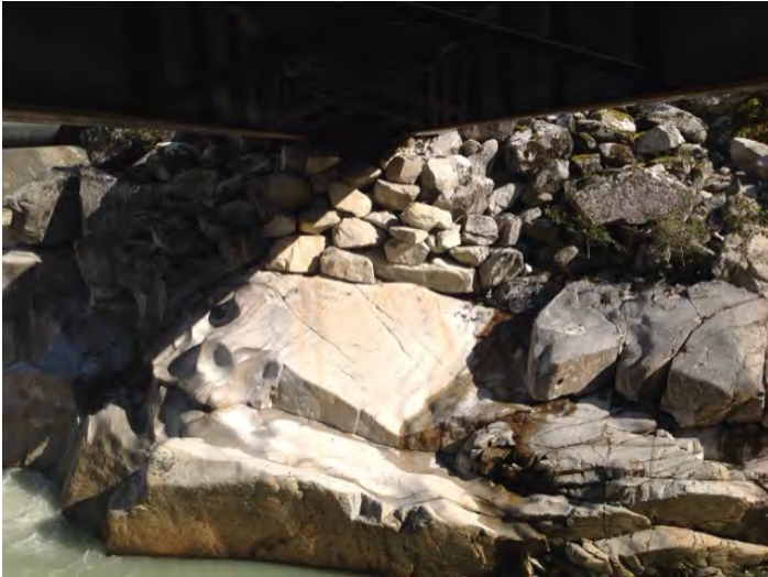
Left Bank Abutment when facing downstream
